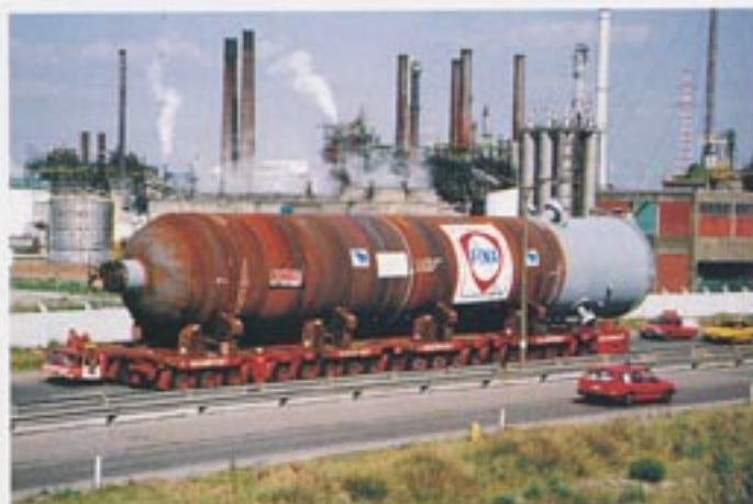
The four heaviest reactors were constructed in Japan. They are 21 meters high and their walls are 30 centimetres thick. To move the heavyweights from the quay to the refinery, Mammoet utilized their SPMTs.
